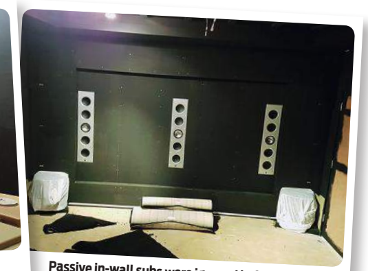
Passive in-wall subs were ignored in favour of two active, sealed SVS SB13-Ultra models. Both were eventually concealed in the front wall
